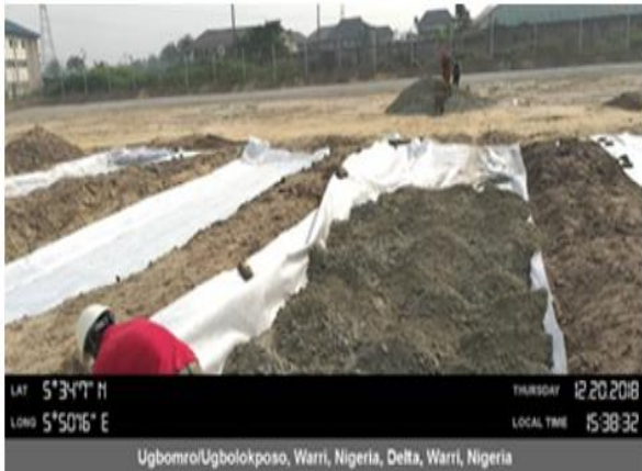
Equipment Foundation Works
