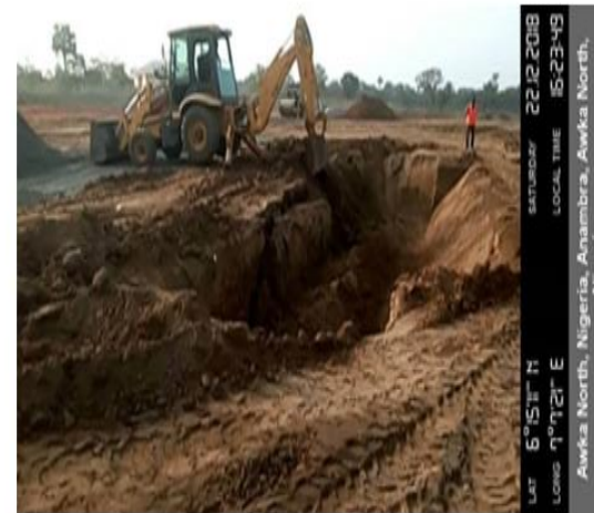
Equipment Foundation Work
