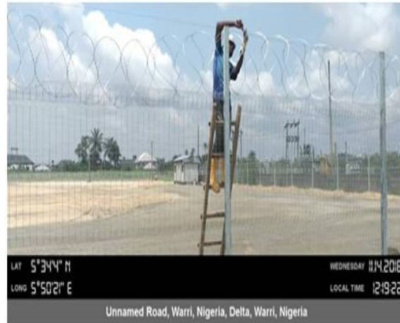
Installation of concertina wire on project site fence (Fencing Completed)
