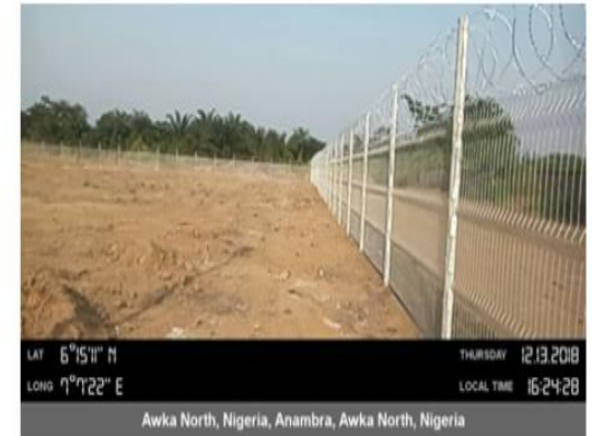
After Site Preparation (Fencing Completed)
