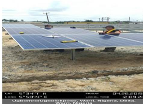
Solar Panels being mounted
