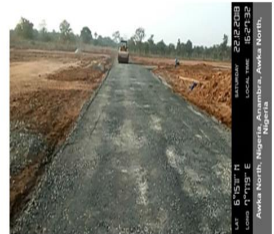
Internal Road Preparation
